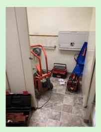
To clear a clog and visually inspect the sewer pipe, both snake and camera were used from the women's restroom. The culprit? A wooden stick and a granite rock someone dropped down the sewer cleanout pipe 75 feet away from the toilet, out by the big birch tree. The broken cap on that pipe has been repaired and a picnic table now sits over the access to keep it less noticeable and minimize a trip hazard.
